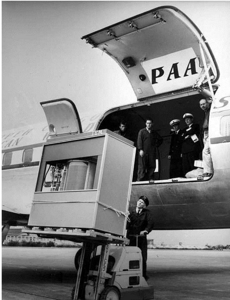
In September 1956 IBM launched the 305 RAMAC, the first 'SUPER' computer with a hard disk drive. The drive weighed over a ton and stored 5 MB of data.
